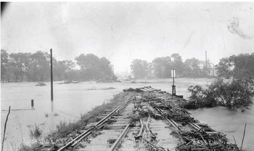
"Looking East From 8th Street"
